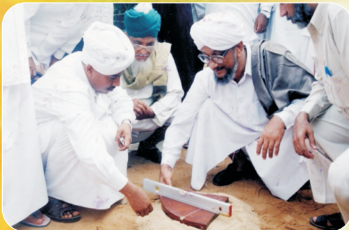
Foundation to Masjid Al Ansar 15/11/2001
